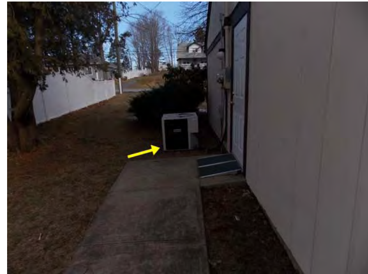
This is the air-cooled condenser, part of the split air conditioning system.
