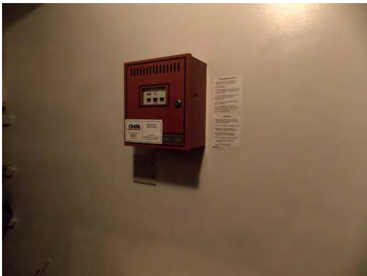
This is the fire alarm control panel.
