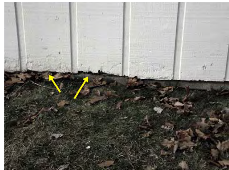
A close-up of isolated deterioration of the wood siding.
