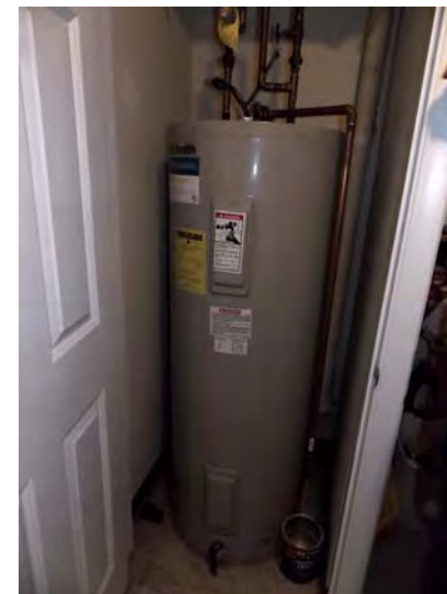
This electric heated DHW tank serves the entire facility.
