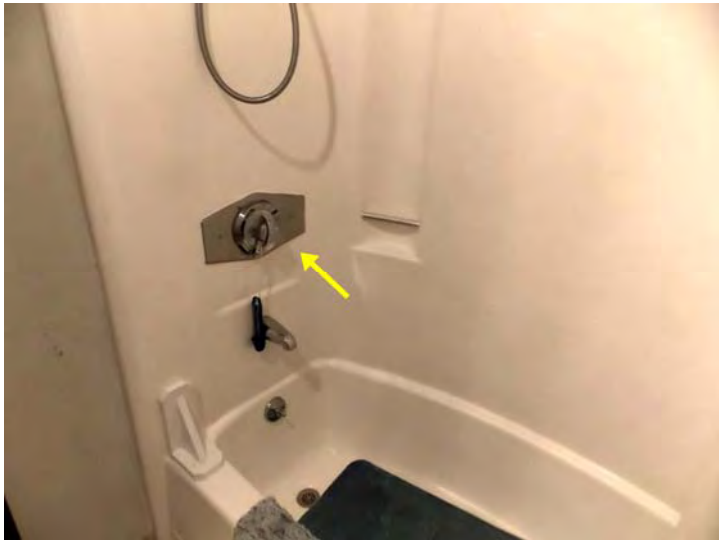
The standard bathroom has a fiberglass tub and tub surround. It also features an anti-scald mixing valve (arrow).
